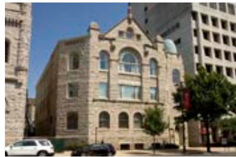
2020–2021 Barrack chilled water plant optimization project completed.
