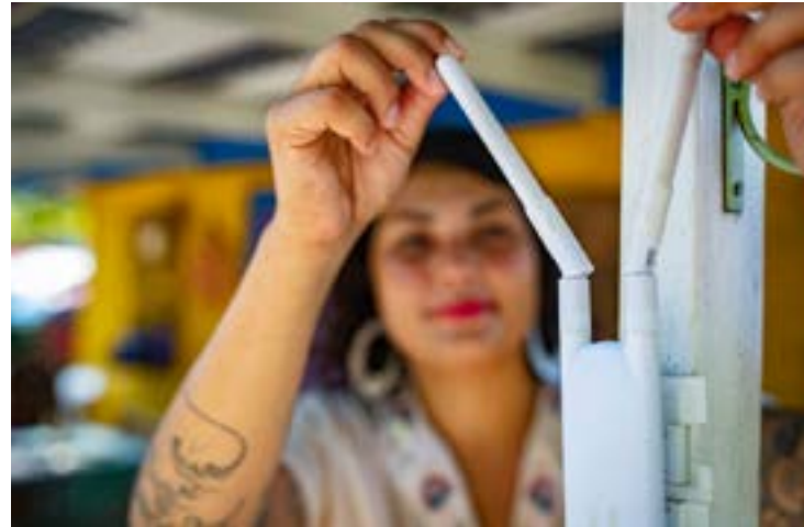
Philly Community Wireless uses mesh networks, in which a collection of nodes act as a single network and antennas pass signals across rooftops, then down to routers, enabling people to connect to the internet for free.
